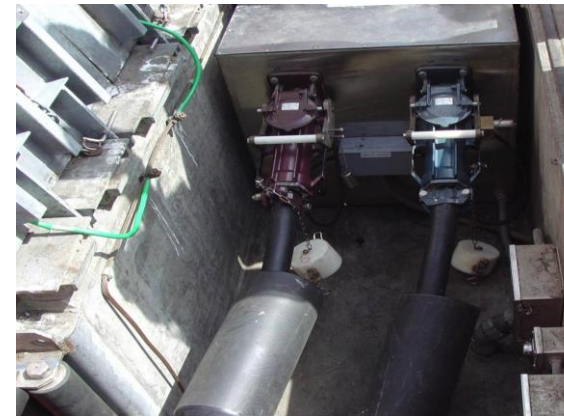
Shoreside Shore Power Outlet connection
