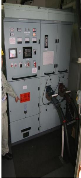
Vessel on-board connection point
