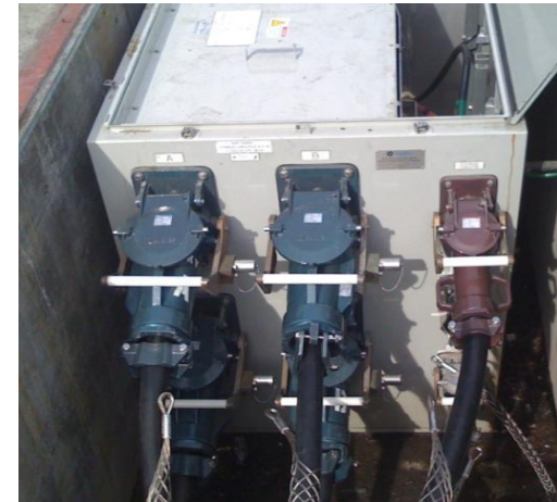
Shoreside shore power outlet connection point
