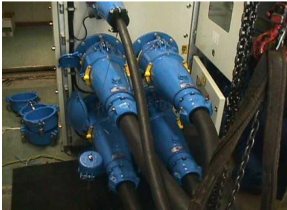
on-board shore power connection point
